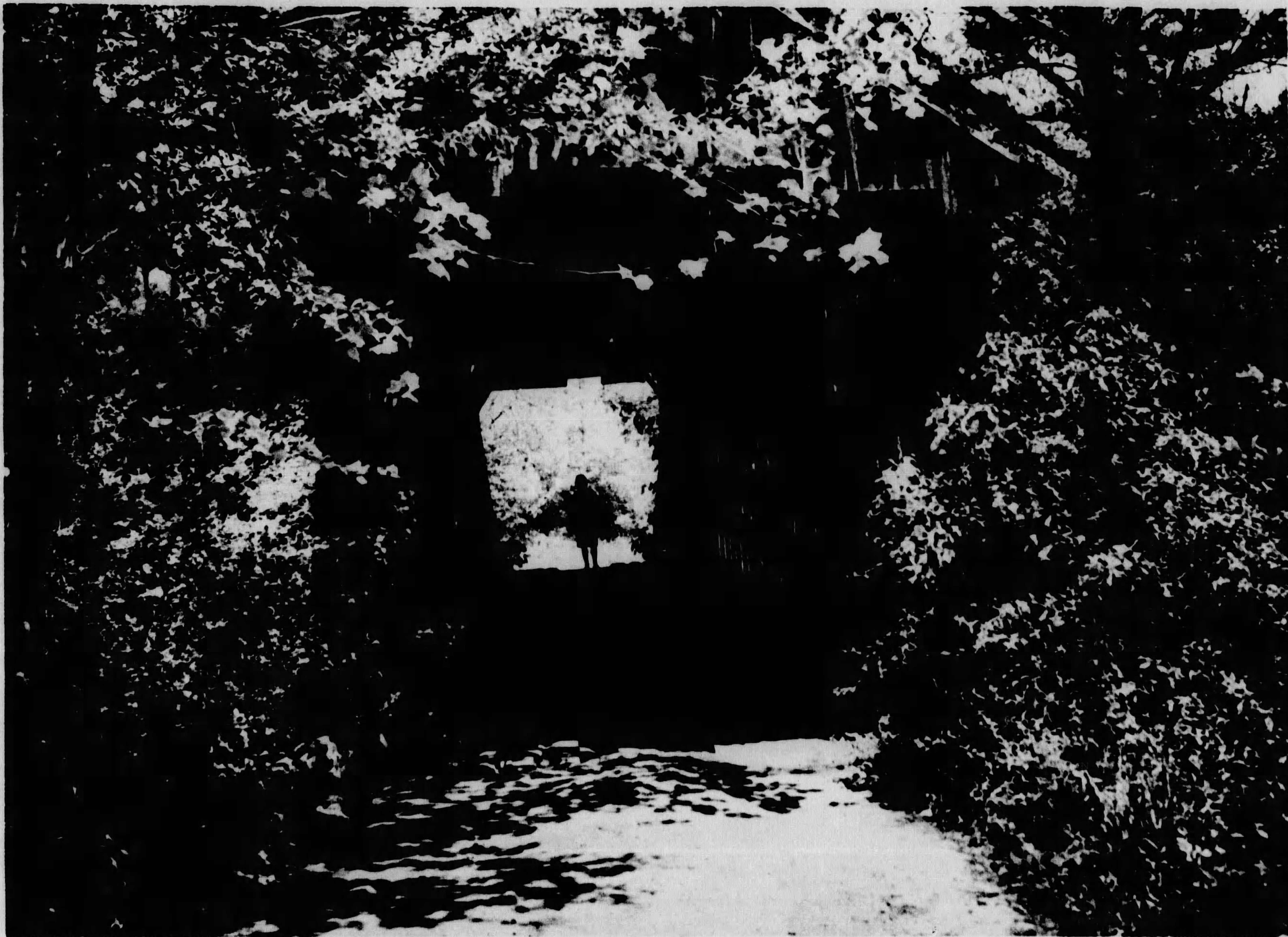
In Forsyth County near Frogtown an old covered bridge crosses a stream which may predict the bridge's future: Settingdown Creek.
